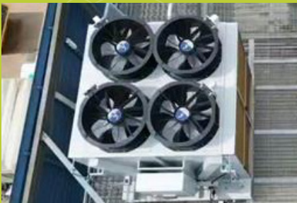
Installation of new CO2 refrigeration system to replace old ammonia systems at our Nottingham site
