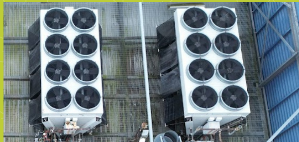
Installation of new CO2 refrigeration system to replace old ammonia systems at our Nottingham site
